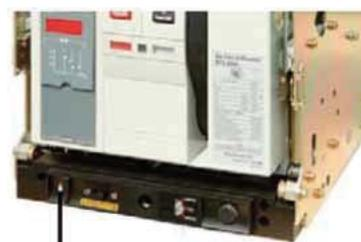
Safety padlock mechanism at the position of "separated"
